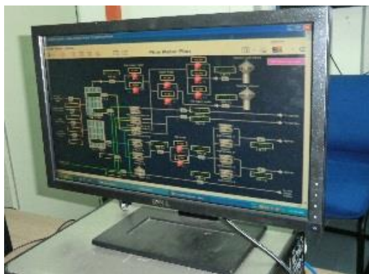
▲ Monitor of SCADA (image)
