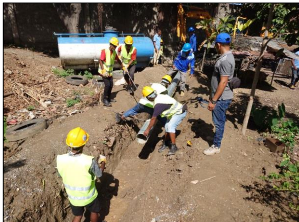
Installment of water distribution pipes
