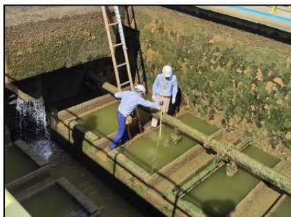
Field survey (Thailand)
