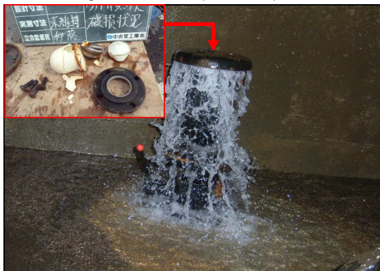
Damage to Air valves on distribution main
