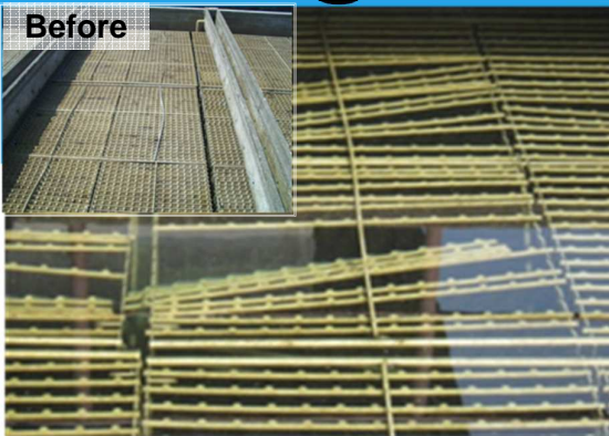
Damage to the tilted plates in plate settler
