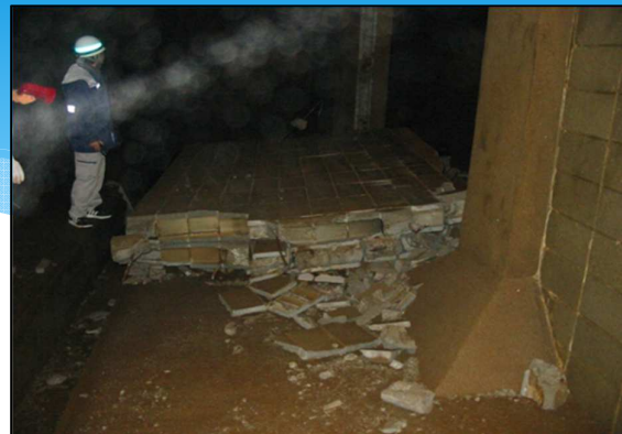
Collapse of flow arrangement wall(Anyoji Reservoir)
