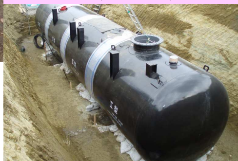
Emergency drinking water storage tank (21 locations)
