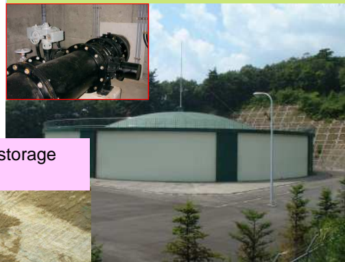
Water reservoir outfitted with Emergency stop valves (20 locations)
