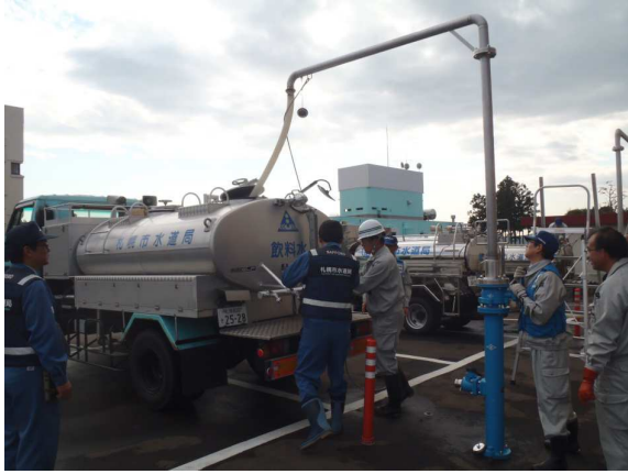
Water replenishment station(Moniwa Plant)
