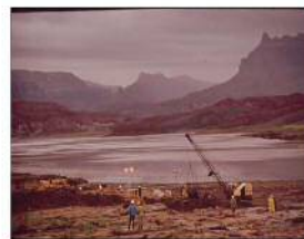
Flood Conditions Caused the Oil and Debris to Spill over Into Nearby Lake Powell. This was contained by a log boom on the Utah side of the border. This View Shows the Boom Site, with Clean Up Equipment in Monument Valley, Utah, 10/1972.
