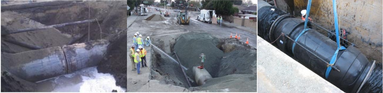
Figure 5. El Portal Main Break/Sinkhole and Mitigation Project Example of Cascading Failures Associated with Collocated Utilities
