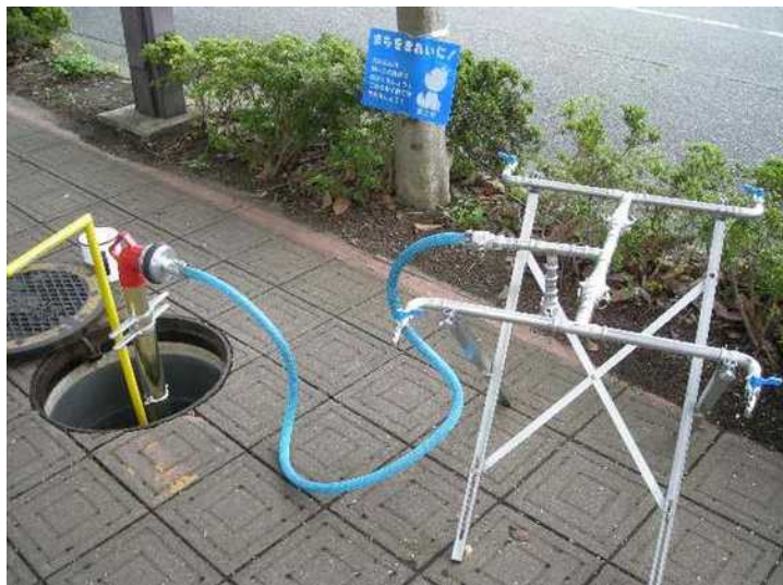
Figure 13. Temporary hydrant
