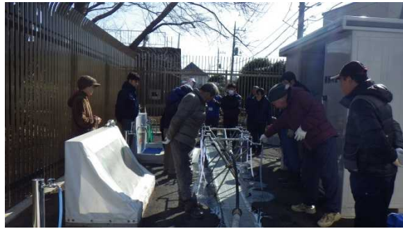
Figure 17. Checking of water flow
