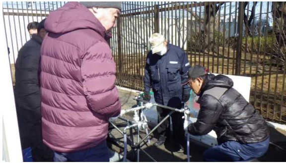
Figure 16. Experience of setting up temporary hydrants
