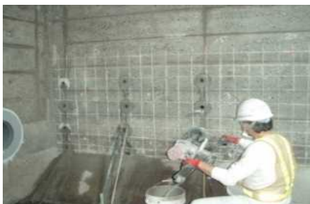
Figure 2. Sidewall boring
