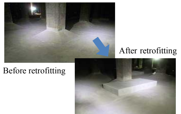
Figure 3. Concrete deck-slab reinforcement
