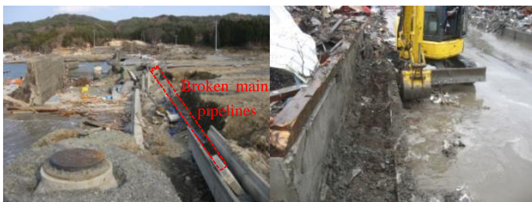
Figure 5 Damage to the pipelines. (left) Broken main pipelines near the coast was washed away and (right) a damaged stop valve with water flowing out.
