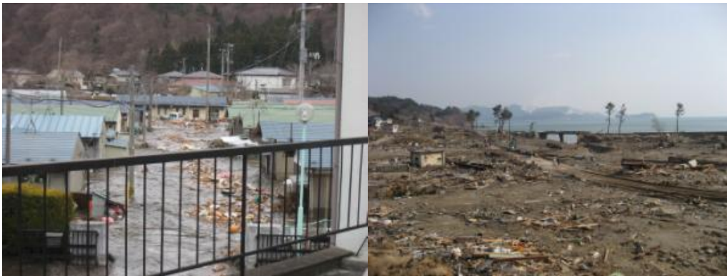
Figure 4 Damage to (left) the water purification plant and (right) the Namiita pumping station .
