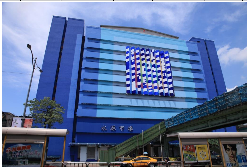
Fig.2 Appearance of Shui Yuan Building
