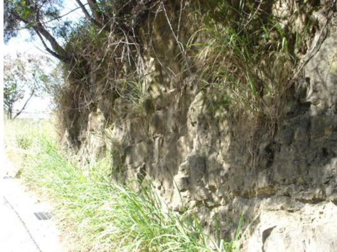
Figure 7 Obvious exposed stratum in the surrounding surface of reservoir.
