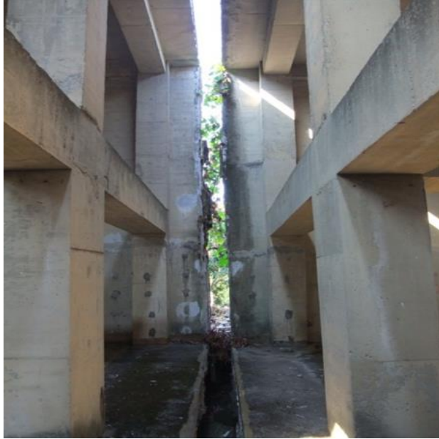
Figure 3 Split of basin from expansion joint
