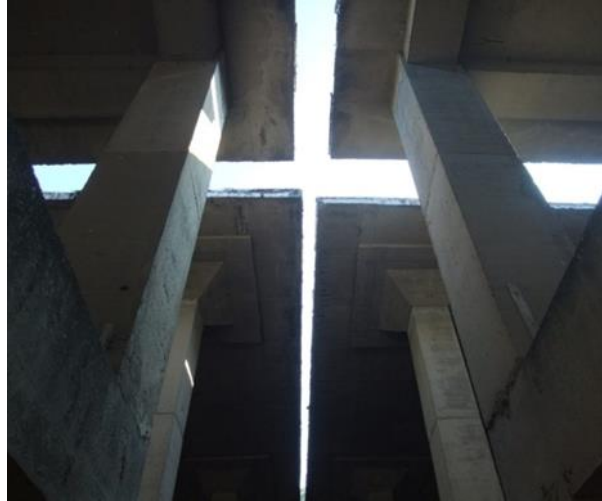
Figure 1 Split of top slab from expansion joint
