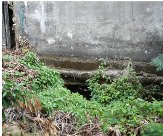
Figure 6 Rupture of ground in the surrounding surface of reservoir.
