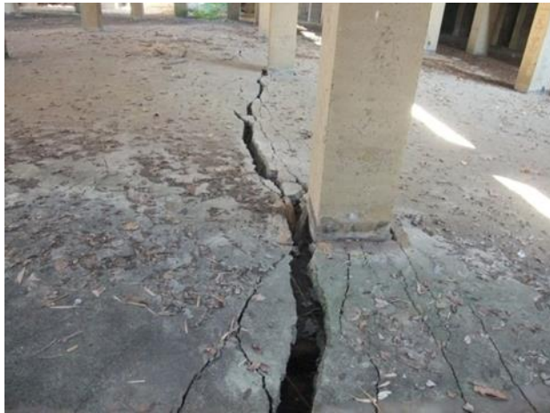
Figure 4 split of bottom slab
