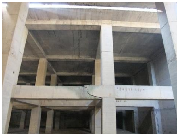
Figure 2 Break in the joint of beam-column joint
